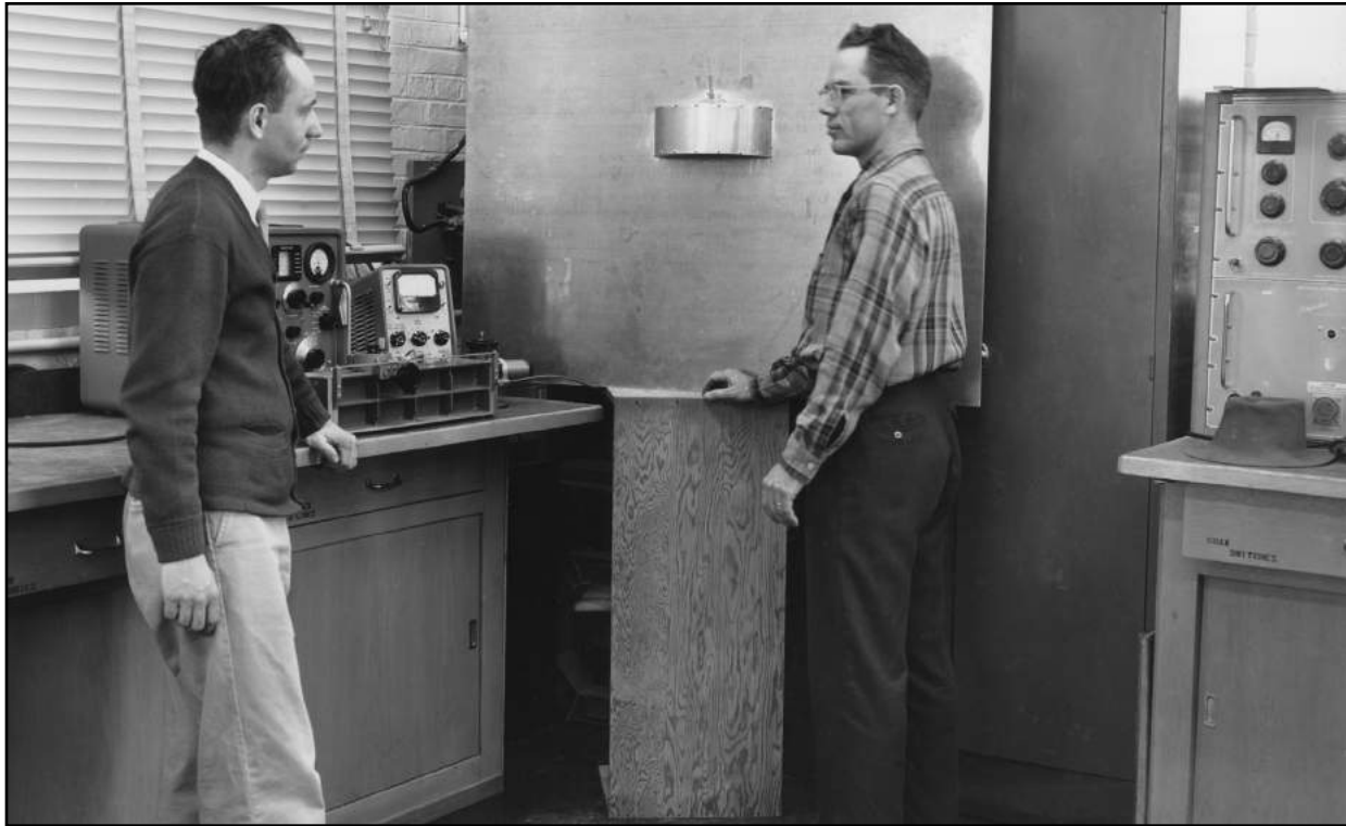
Photo 28-2.4. Author Maxwell with technician John Luzansky (L) viewing the half-shell 1:4 scale model of TIROS 1 mounted on ground plane for obtaining antenna impedance data during development of the antenna system. Note the HP-805 slotted line near Luzansky's left hand, used for obtaining the impedance measurements.
