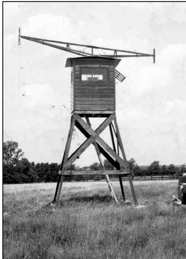
Photo 30-1. The FCC Adcock direction-finding station at Lexington, Kentucky, in 1941. This station is typical of FCC direction-finding Adcocks used at all FCC monitoring stations in the US mainland, Hawaii, Alaska, and Puerto Rico.
