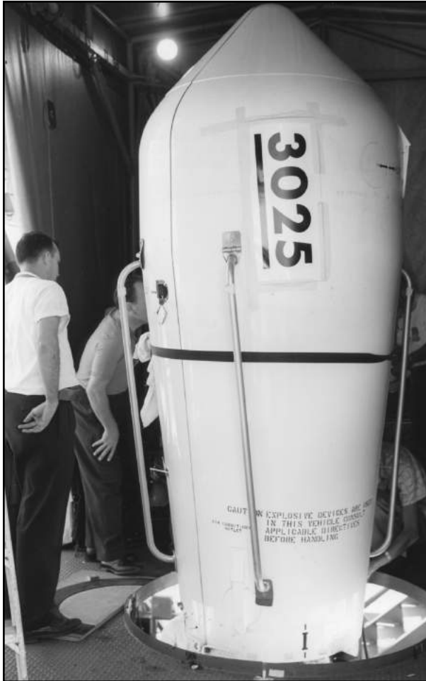
Photo 28-2.17. In this photo the gantry at launch pad 17A is in place around the entire height of the rocket structure and spacecraft. The photo was taken at the top level of the gantry, at the level of the spacecraft as shown in Photo 28-2.10 with the gantry rolled away. The photo shows author Maxwell peering into the fairing, or nose cone, that houses the third-stage booster rocket and the spacecraft. He is inspecting his antennas on the spacecraft atop the rocketry to determine whether the ends of the antennas fit properly into the fairing.
